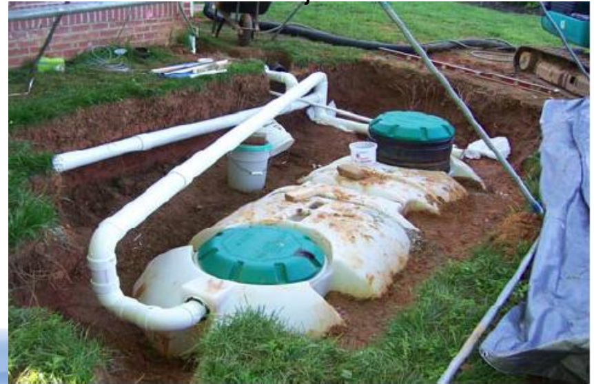
Residential Cistern Project – Installation
