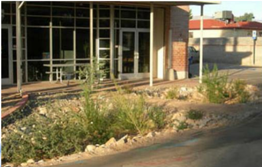
Municipal facility onsite capture.
