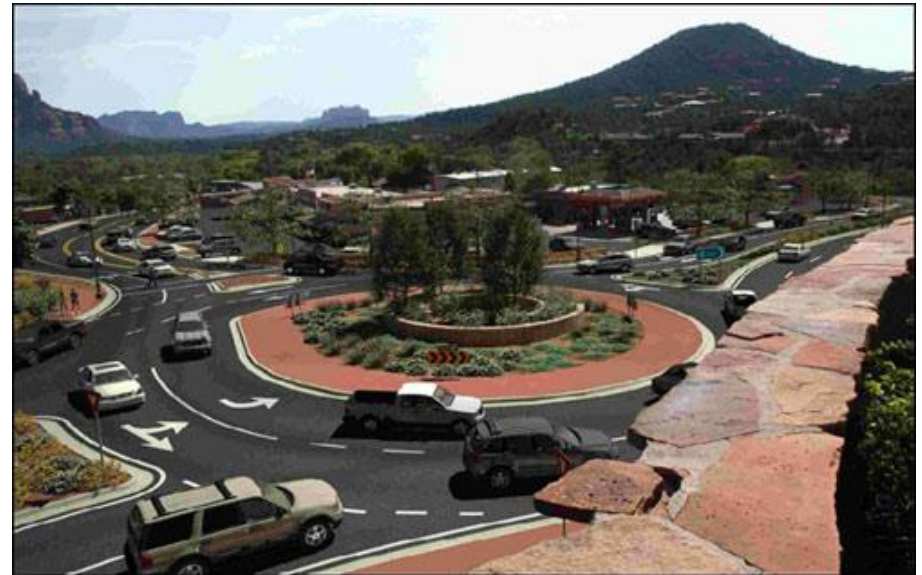
Arizona State Highway 179, Sedona, AZ
