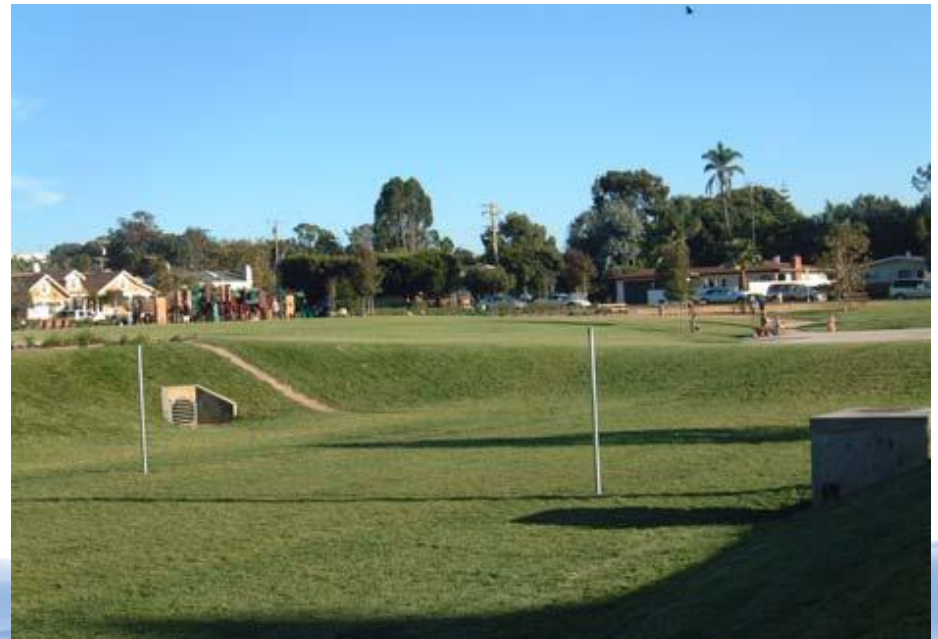
Park stormwater detention basin also serving as playing field.
