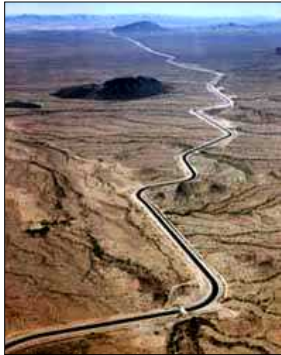
Central Arizona Project (CAP) Colorado River (43-45%)
