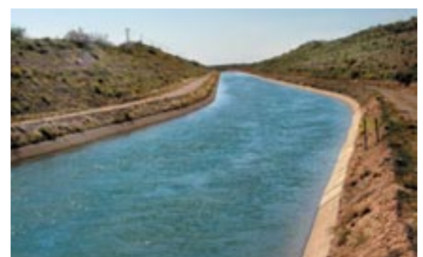
Central Arizona Project, near Florence
