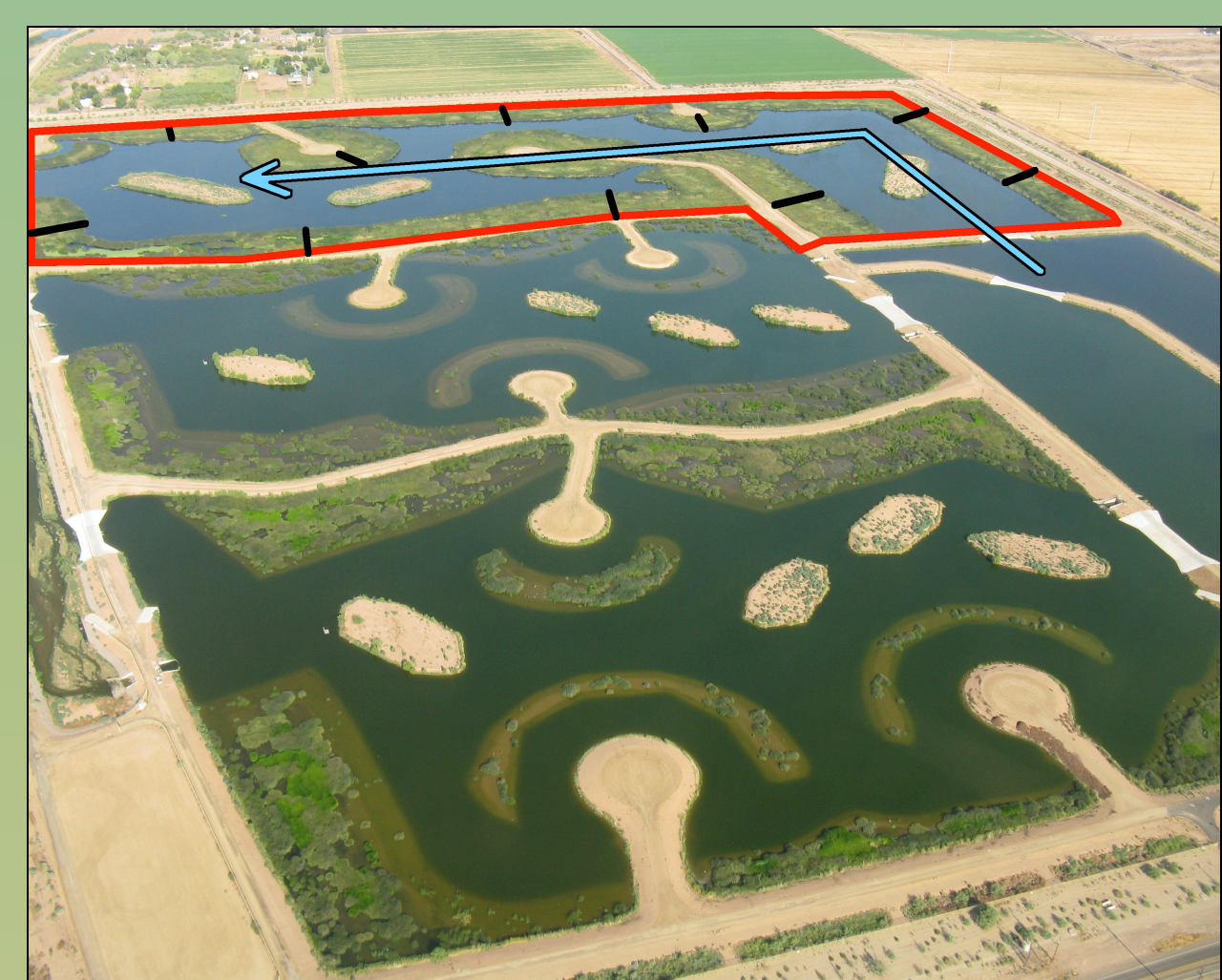
Figure 1A: Aerial photo of the treatment flow cell
