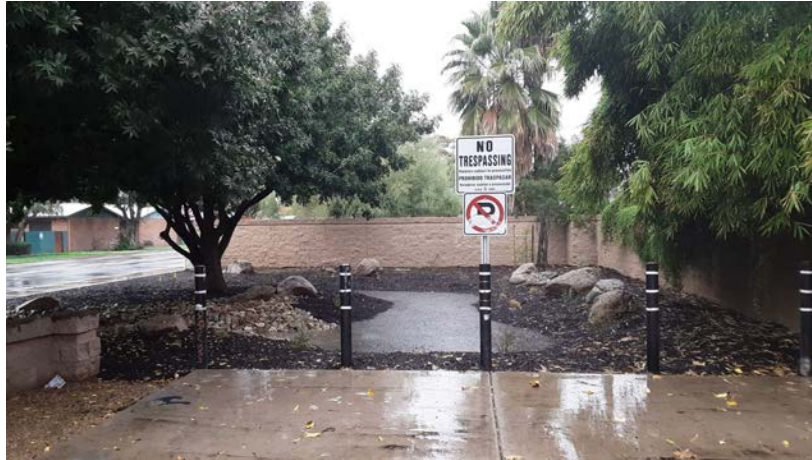
Figure 12: Green infrastructure - Bioswales are one example of green infrastructure that provide localized cooling solutions and harvest stormwater. Picture credit: City of Tempe
